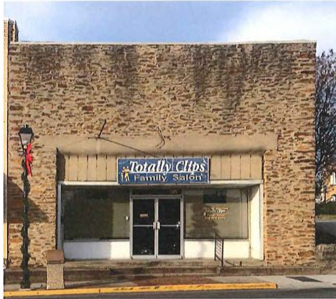
Existing Front Facade
