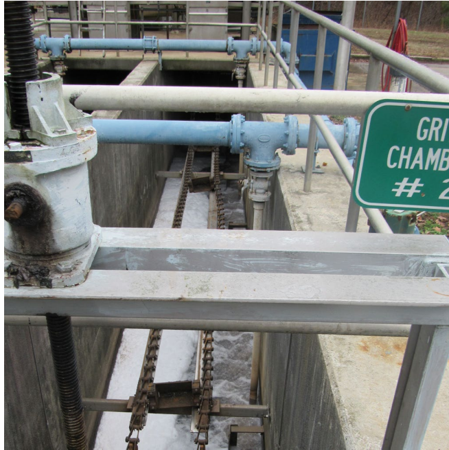
Replace Grit Removal System – Wastewater Treatment Plant
