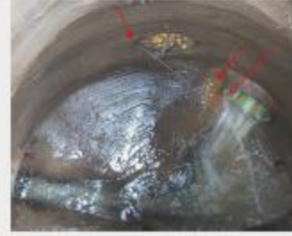
MANHOLES WITH ACTIVE LEAKS
