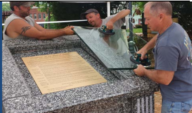
The six documents will be original size on 1/4" etched bronze. Each document weighs over 60 pounds and covered by engineered industrial viewing glass.
