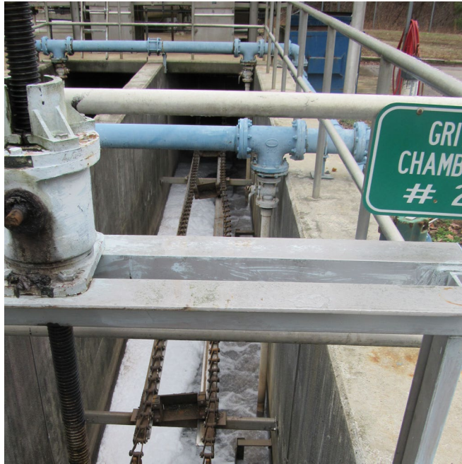
Replace Grit Removal System – Wastewater Treatment Plant
